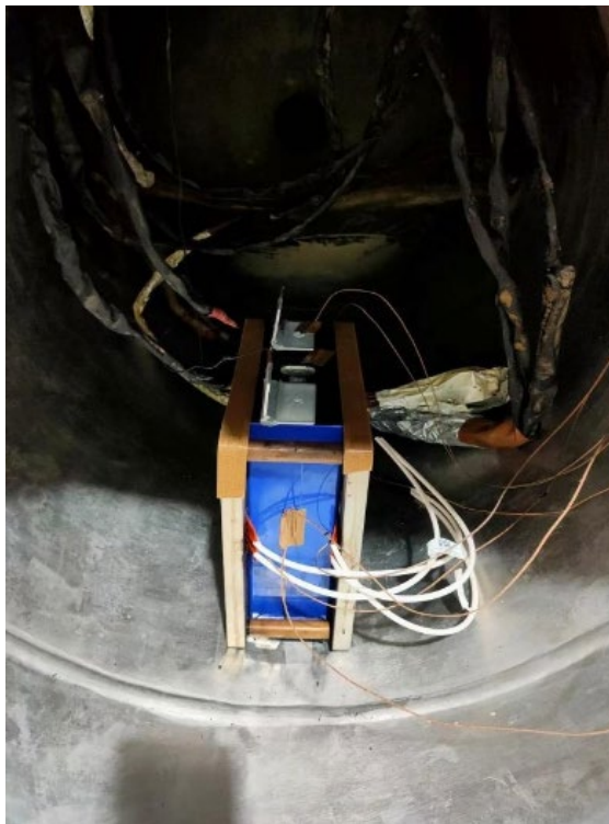
Figure 7. Battery Gas Composition Test Chamber
